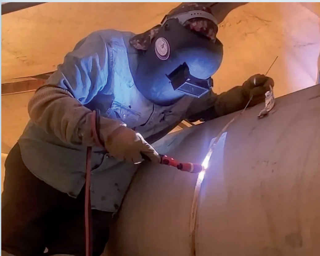
Field GTAW welding of 304H stainless piping during fabrication of a high-temperature process system.
